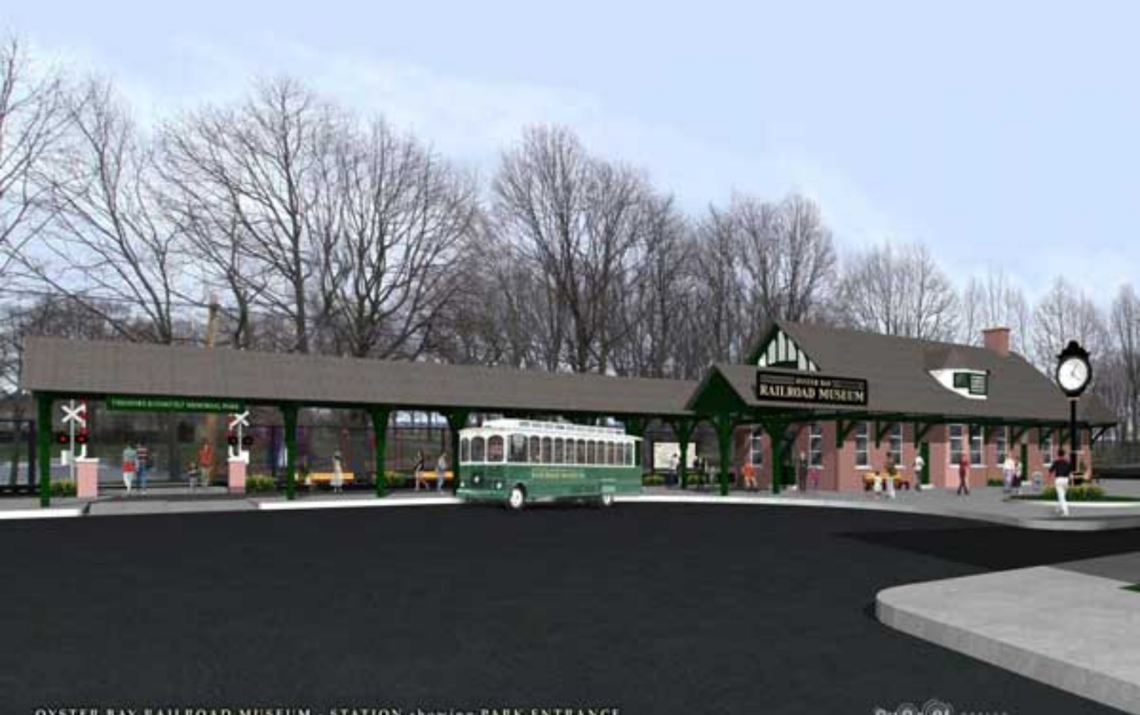
OYSTER BAY RAILROAD MUSEUM - STATION showing PARK ENTRANCE
