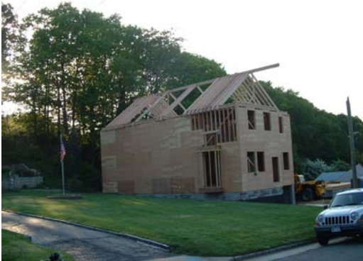
124 Summers Street ▪ Under Construction (Demolition/Subdivision) Lot Size : 7,867 SF GFA : 3.230 SF / 2.873 SF
