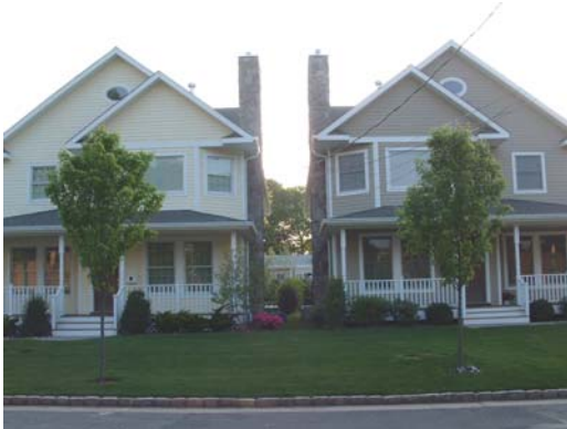
156 Summers Street (Left) ▪ Built 2004 (Demolition/Subdivision) Lot Size : 7,575 SF GFA : 3,728 SF / 2,815 SF
