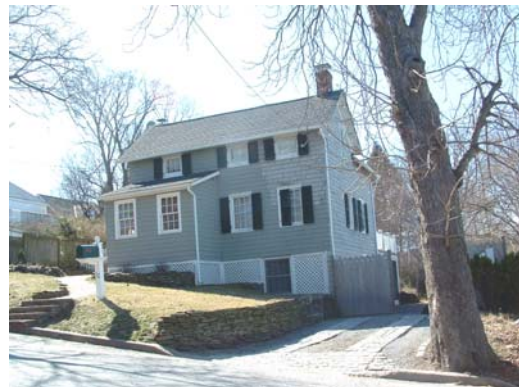
12 Prospect Street • Built 1838 (Historic Landmark) Lot Size : 5,512 SF GFA : 1,284 SF / 2,205 SF
