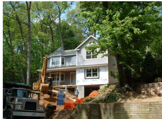
McCouns Lane ▪ Under Construction Lot Size : 4,356 SF GFA : 2,650 SF / 1,742 SF
