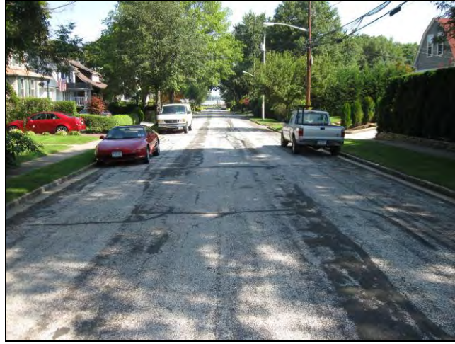
Views of Ships Point Lane residences, which is a potential candidate for a green streets retrofit.
