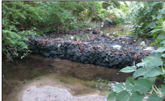
Gabion wall along reach CSB-04
