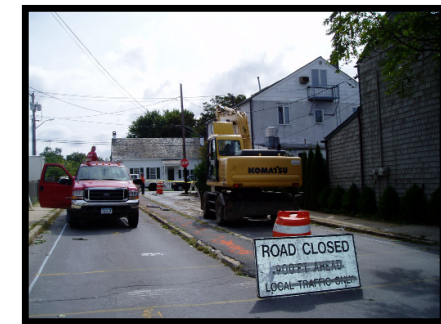
Townsend Square Parking Lot (before)
