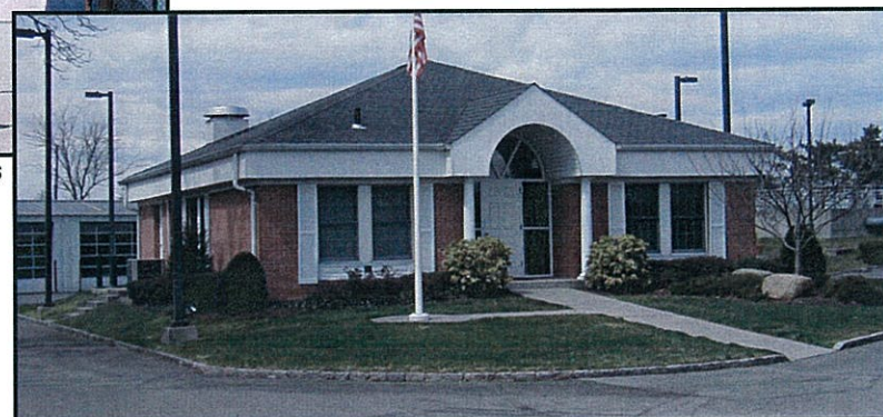
Sewage Treatment Plant
