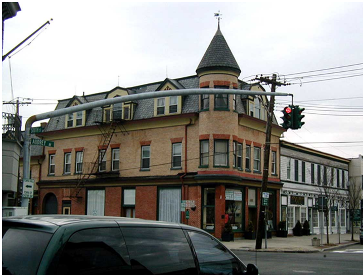
The photo above shows a jumble of overhead wires and an unsightly pole. In addition to their esthetic appeal, underground utilities are more reliable and less costly to maintain. The photo at the right is a simulated view after removal of overhead wires.
