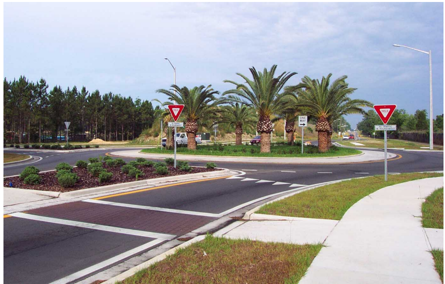
Larger roundabouts, such as this example from Gainsville, Florida, may require right-of-way acquisition. Many variables influence the diameter of the roundabout, including the type and size of vehicles that must be accommodated. The photo and the drawing above show the effective use of splitter islands, the triangular island at the entry to the roundabout. Note that crosswalks are set back from the entry point of the roundabout.
