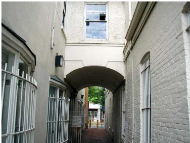
Beautification efforts, such as repairing broken windows, painting, and general clean up can yield benefits much larger than the effort invested.
