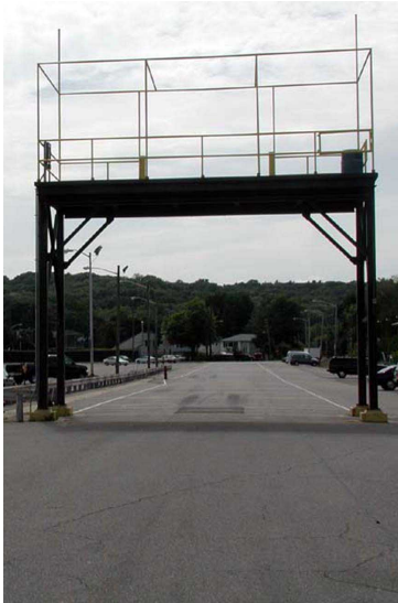
Training tower at Firemen's Field. This site has been used for competitive training activities by firemen for many years. Those activities need not be precluded by the addition of housing units and a new parking lot configuration. The area can accommodate all uses and also be much more aesthetically pleasing.
