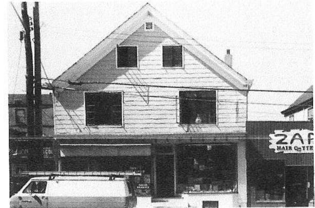
Typical existing facade on South Street.
