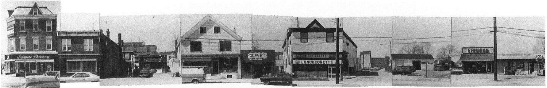
West side of South Street above Audrey Avenue, today.
