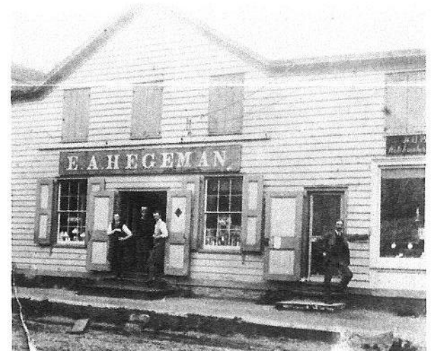
Grocery store at site of present Bank of North America.
