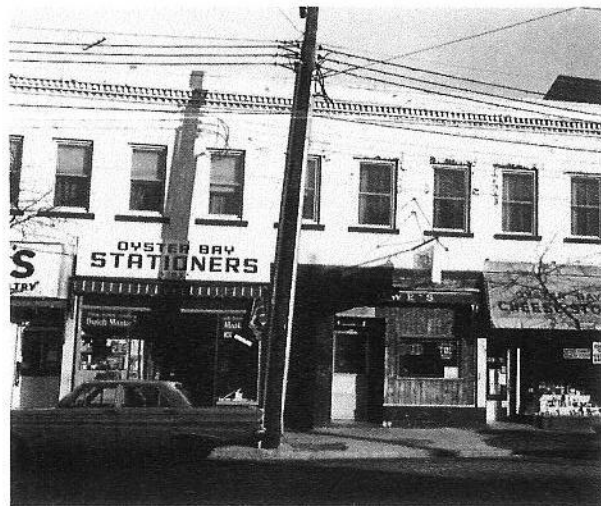
Uncoordinated facades on South street today.
